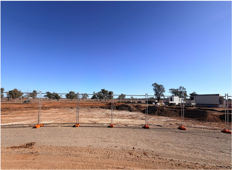
Early earthworks for ne Skin Shed
