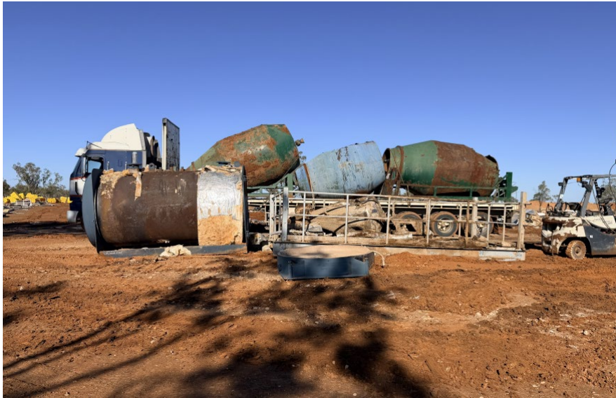
Metal recycling activity in laydown yard
