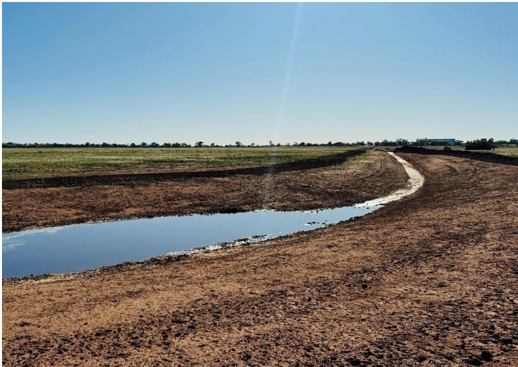
Figure 13: Tail-water Pond and Swale Drain
