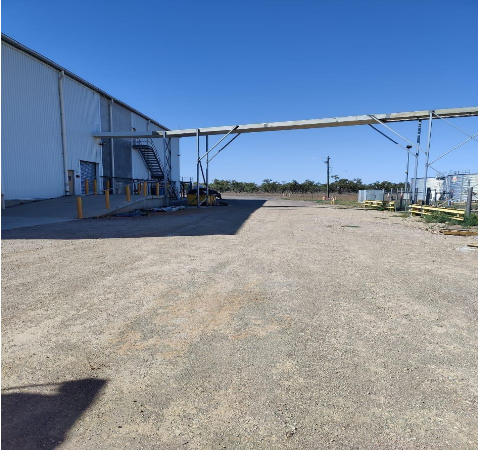
Figure 3: Rear side road of the building
