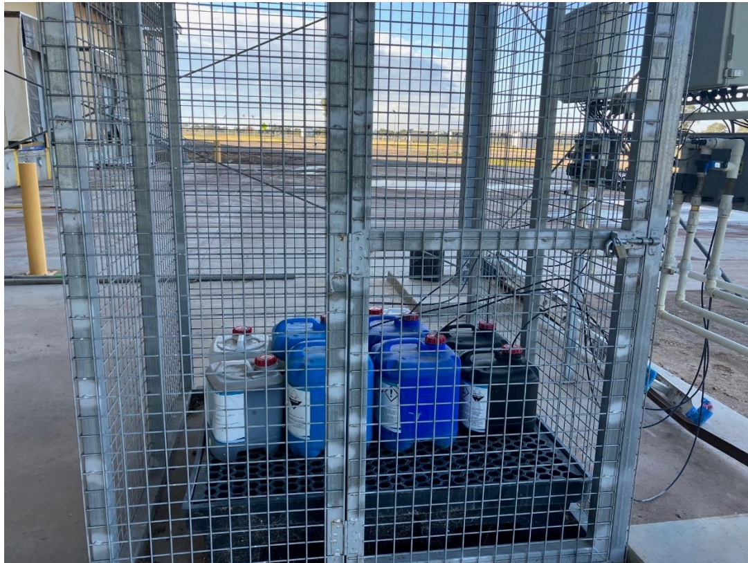
Figure 9: Water dosing chemical stored on a bunding
