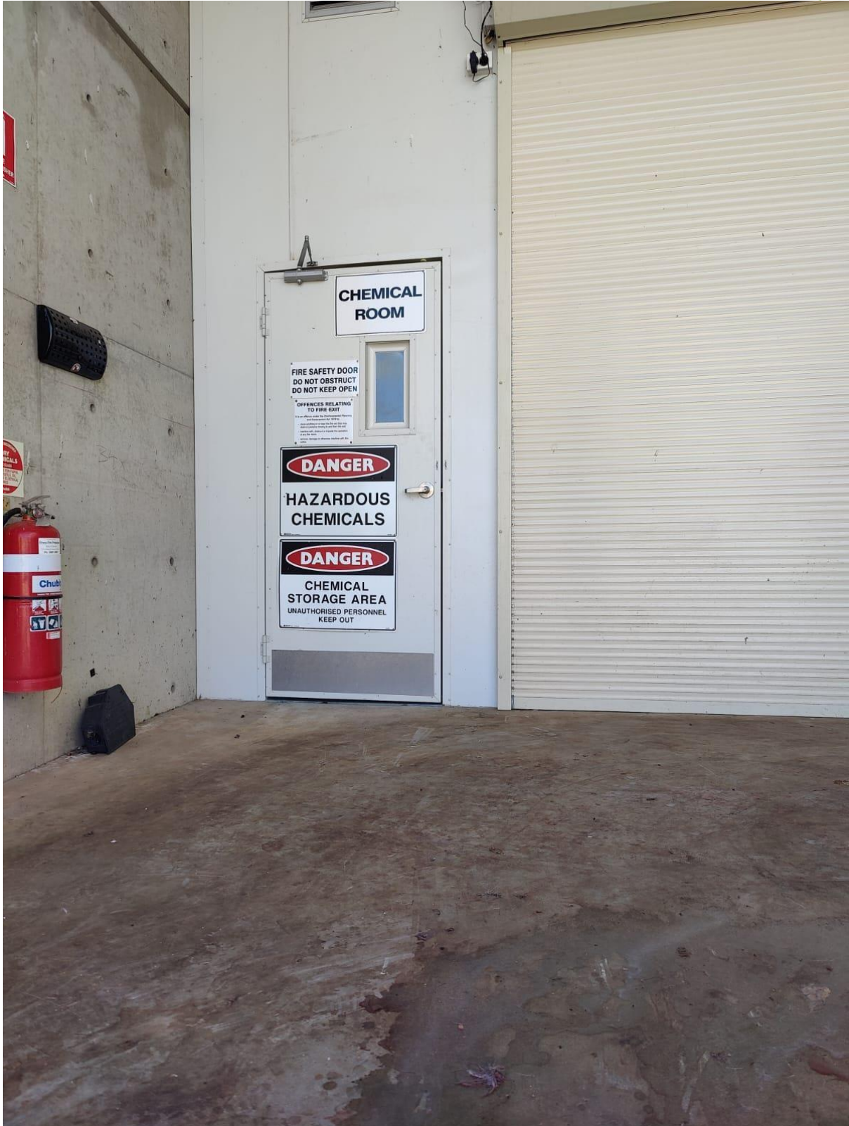
Figure 13: Chemical Room Signage (a)
