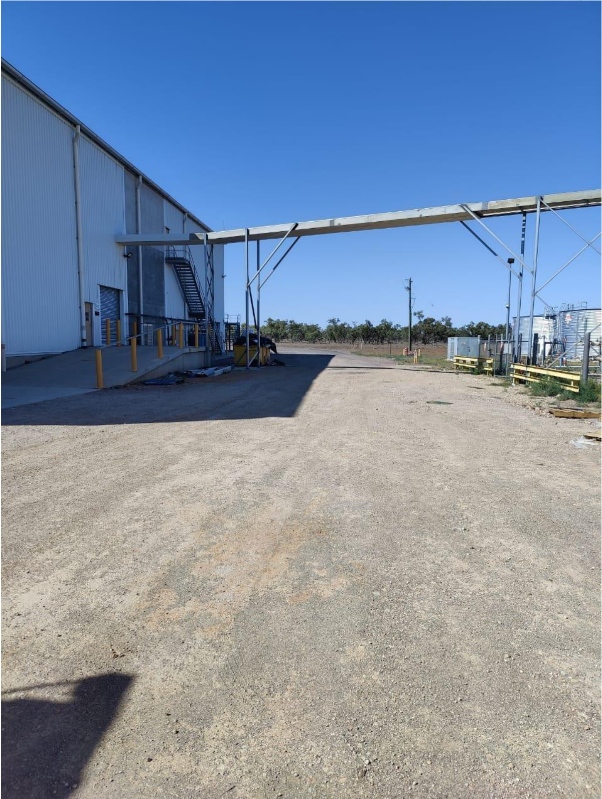
Figure 4: Backside road of the building
