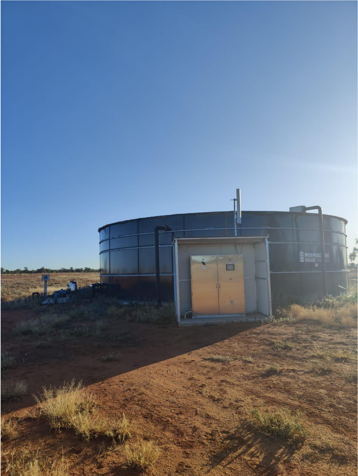
Figure 16: Balance Tank in WWTP Area
