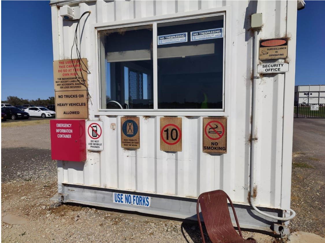
Figure 6: Security office at front entrance
