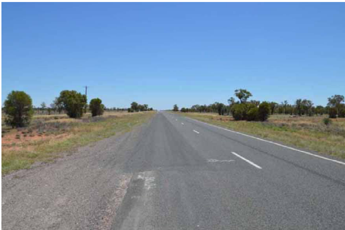
Photograph 2.2 The Mitchell Highway in the vicinity of the project site access, looking north
